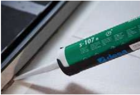
10- Edge joints occurring at corners, changes of paving level and changes of material should be covered with tile trim or a tile itself and sealed with flexible sealant. Minimum joint width: 8 mm.
