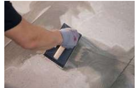
15- Follow the manufacturer's recommendations in respect of the preparation and use of grouting materials. Ensure that the material and tools chosen do not damage the tile surface. The grout should be applied using a rubber trowel. VENIS catalogues contain details of the butech materials recommended for each design.
