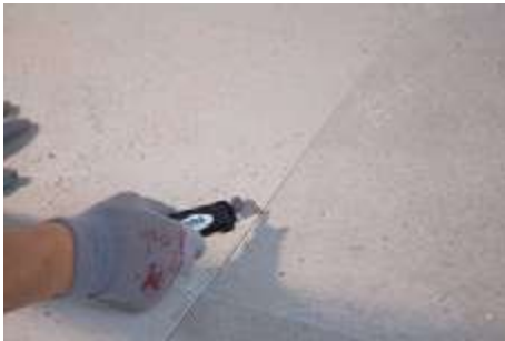
13- Prior to grouting, check that the bonding material has hardened. Remove the tile spacers, clean the joints along their length, width and depth, and check the joint is not damp.
