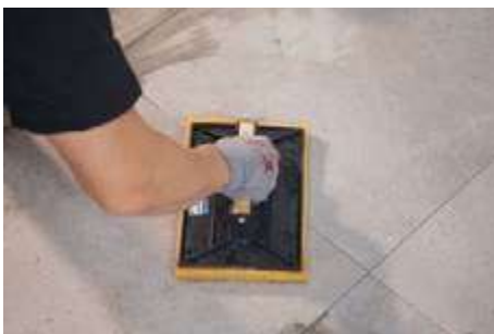
16- Wait for the grout to start to dry, then clean with a sponge dampened in clean water. Do not allow the grout to harden on the tile, especially on textured tiles. Do not soak the joint with excess water.
